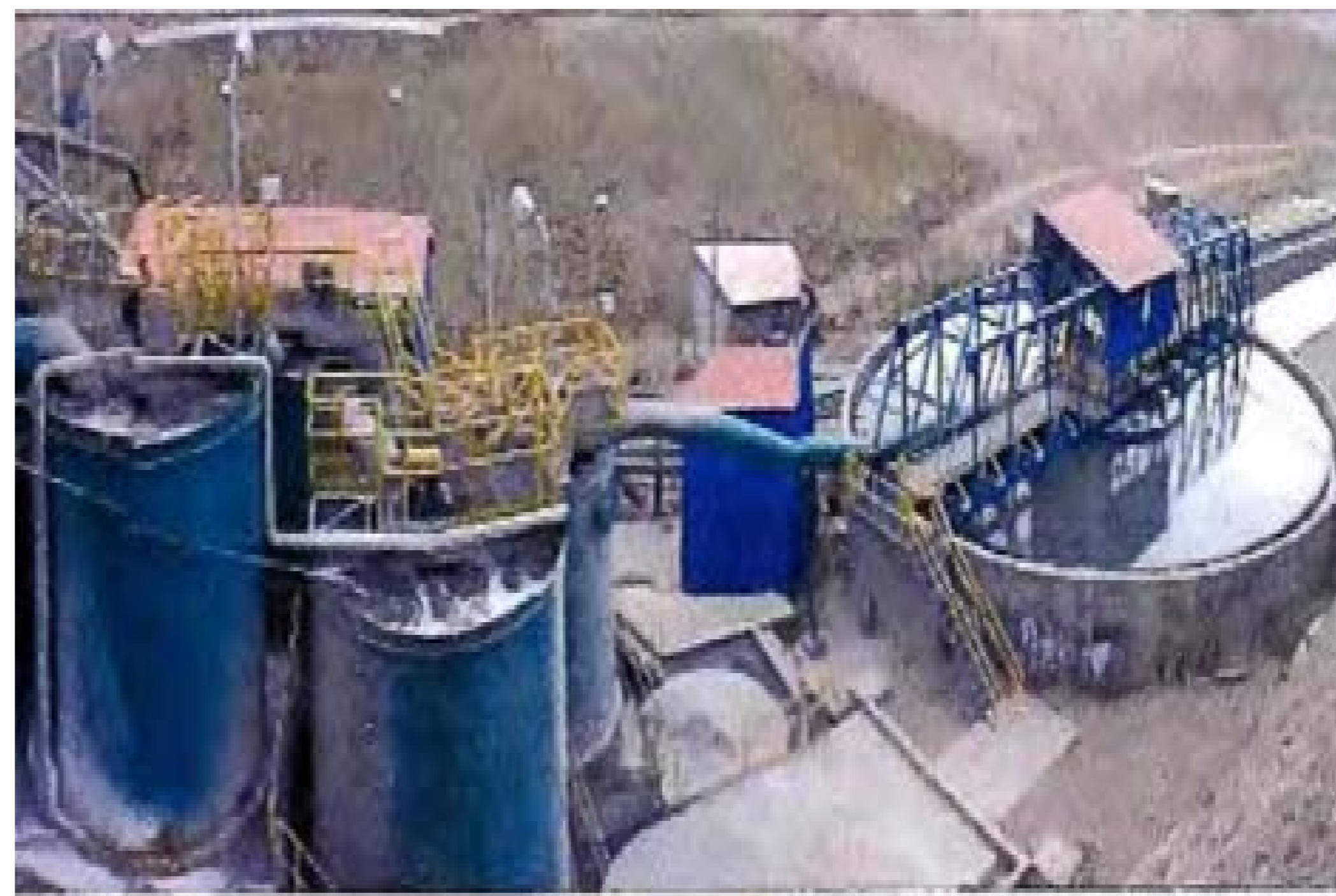
Mining effluent treatment plant : NCD process
